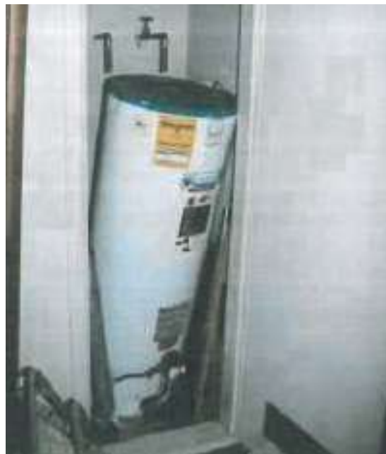
Photo of water heater failure in 1994 Northridge Earthquake. COURTESY OF EXPONENT
