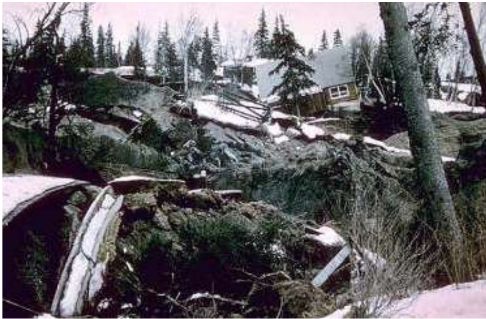
The Turnagain Heights landslide in Anchorage, Alaska. Seventy-five homes twisted, slumped, or collapsed when liquefaction of subsoils caused parts of the suburban bluff to move as much as 2,000 feet downward toward the bay, forming a complex system of ridges and depressions. The slide developed because of a loss in strength of the soils, particularly of lenses of sand, that underlay the slide.
