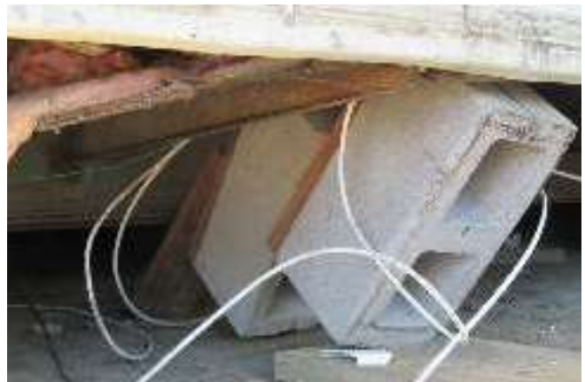
Manufactured home rotated and fallen support piers.
