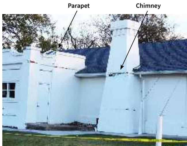
Masonry parapet separation.
