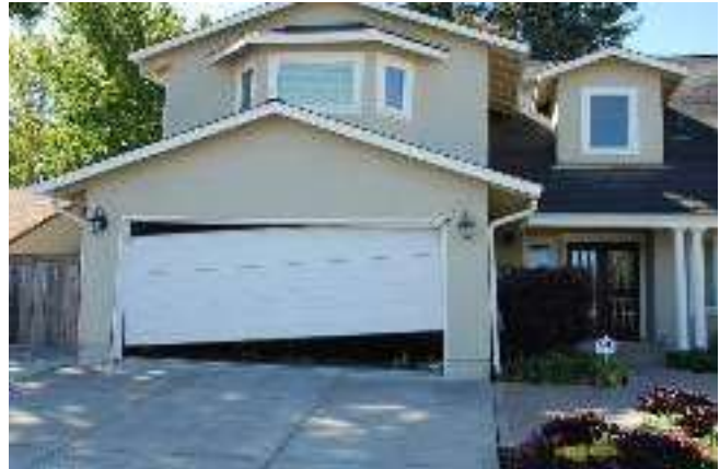
Examples of significant earthquake damage—portions of homes that appear to be leaning or have fallen down.
