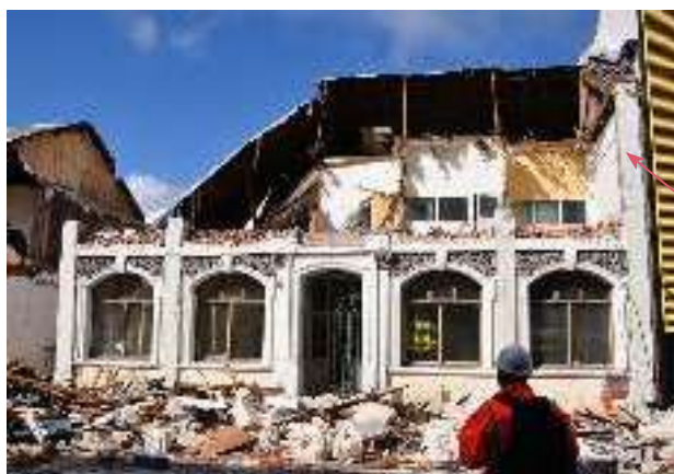
Photo of damage to masonry building in Christchurch. COURTESY OF FRED TURNER, AVAILABLE AT WWW.EERI.ORG, LAST ACCESSED 8/3/19
