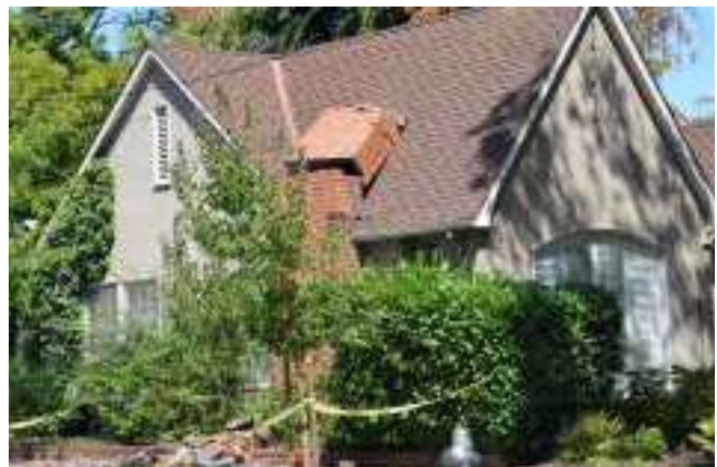
Earthquake damaged chimney.
