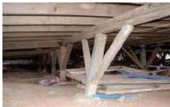
Photo of damage to post and piers in Hawaii Earthquake. COURTESY OF IAN ROBERTSON, AVAILABLE AT WWW.EERI.ORG, LAST ACCESSED 7/7/19
