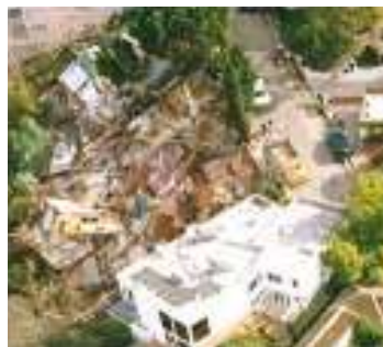
Hillside homes collapsed in the 1994 Northridge Earthquake. PHOTO COURTESY OF CITY OF LOS ANGELES DEPARTMENT OF BUILDING AND SAFETY
