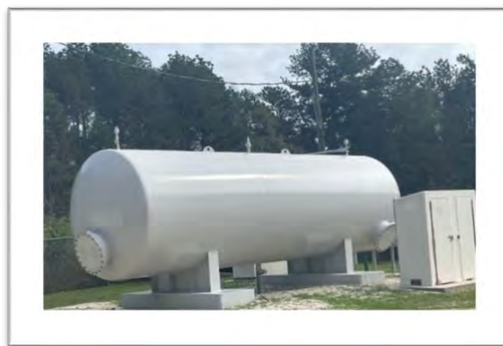
Hydropneumatic Tank Installed
