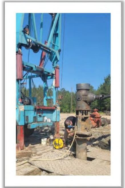
Potable Water Supply Well in Construction
