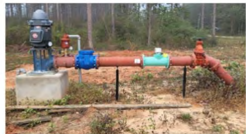
Potable Water Supply Well in Construction
